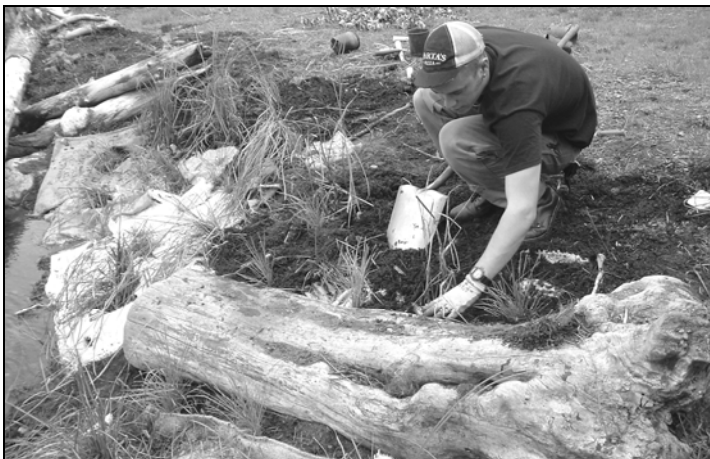
A crew member with EarthCorps installs saltwater-tolerant grasses near the mouth of Fauntleroy Creek.
