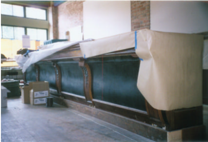
The lower portion of the 20' mahogany bar being installed in Endolyne Joe's
